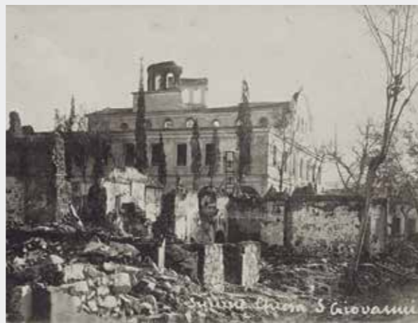
3 Damage to orthodox church, 1922.
